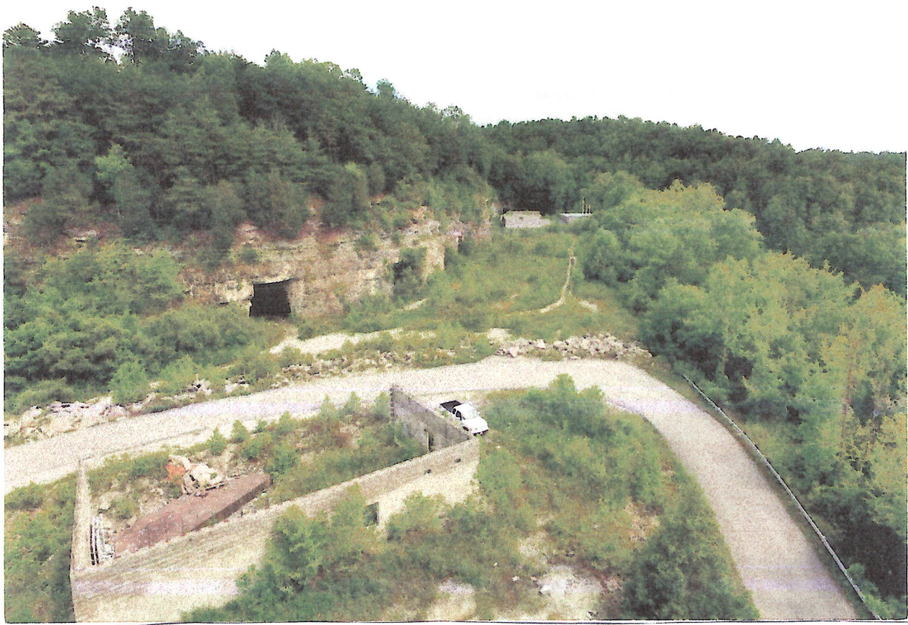
Photo above: Looking along exterior plateau from west to east including the start of one building.
